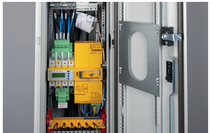
Detail new installation
