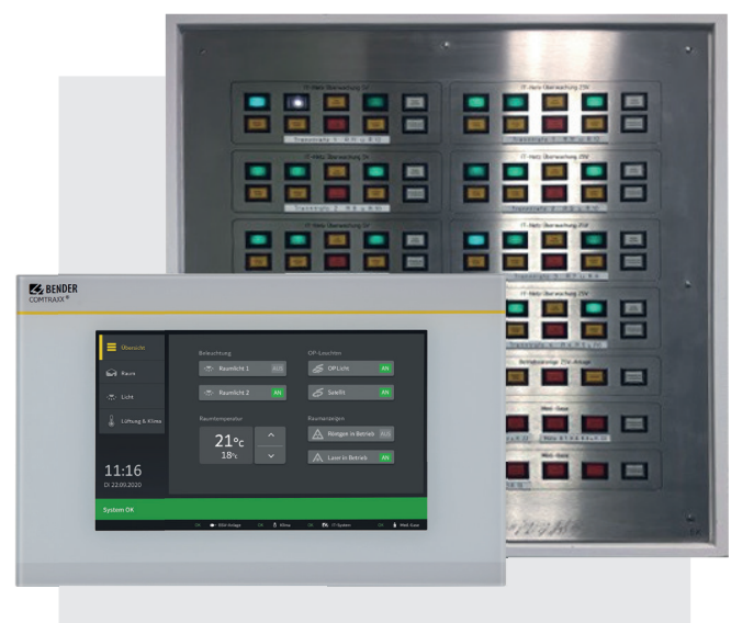
Detail old and new installation
