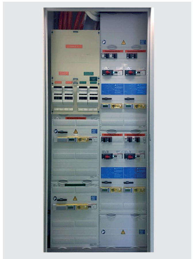
Detail new installation
